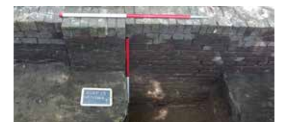
IMAGE FOUR: THE BRICK WALL ADJACENT TO THE GATE HAD BEEN PUSHED OVER AND LEVELLED, BUT BENEATH THE SURFACE WAS IN GOOD CONDITION.
