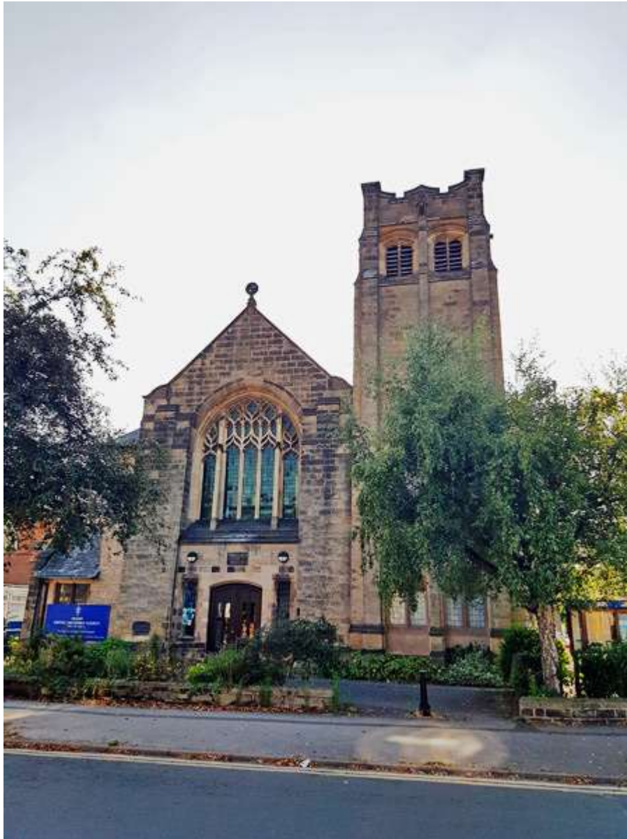
Friary Church, Musters Road, West Bridgford, 2023 (author's photograph)
